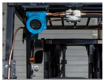
MINERAL INSULATED CABLES designed to meet needs of non-combustible, heat and water resistant cable. Made of highly compressed mineral. The cables are sealed in a seamless copper tube, ensuring safety, making them liquid and gas tight. MI cabling provides flexibility and space saving.
